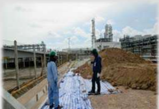
Prevent soil falling to drainage
